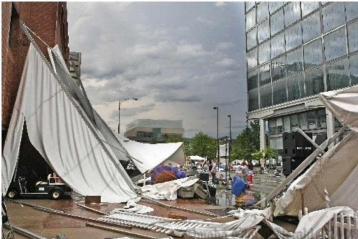
6/27/08 - Aftermath looking North
